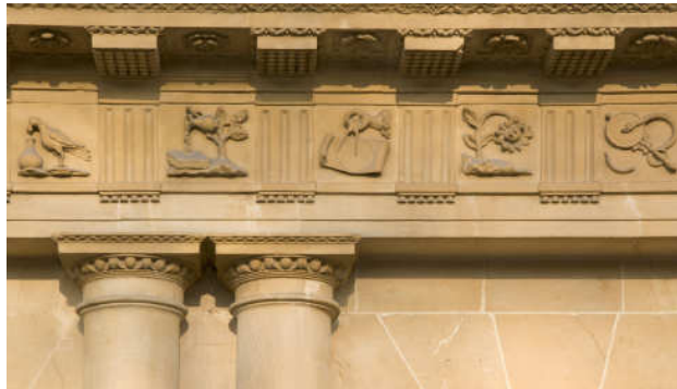
The Circus (Bath), UK. Architectural detail of the frieze showing the alternating triglyphs and metope. (John Wood, the Elder, architect).
